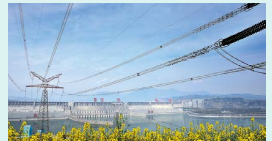
Electricity Transmission Line of Three Gorges HPP
