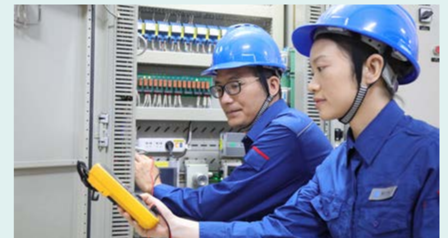
Left-bank power house at Xiangjiaba HPP
